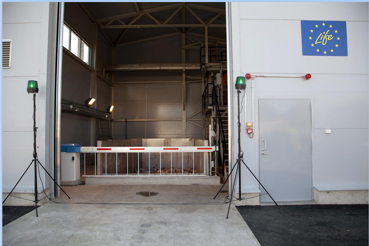
Picture 2. Part of the receiving station building is seen in the picture. The door is open and the safety beam is down.
